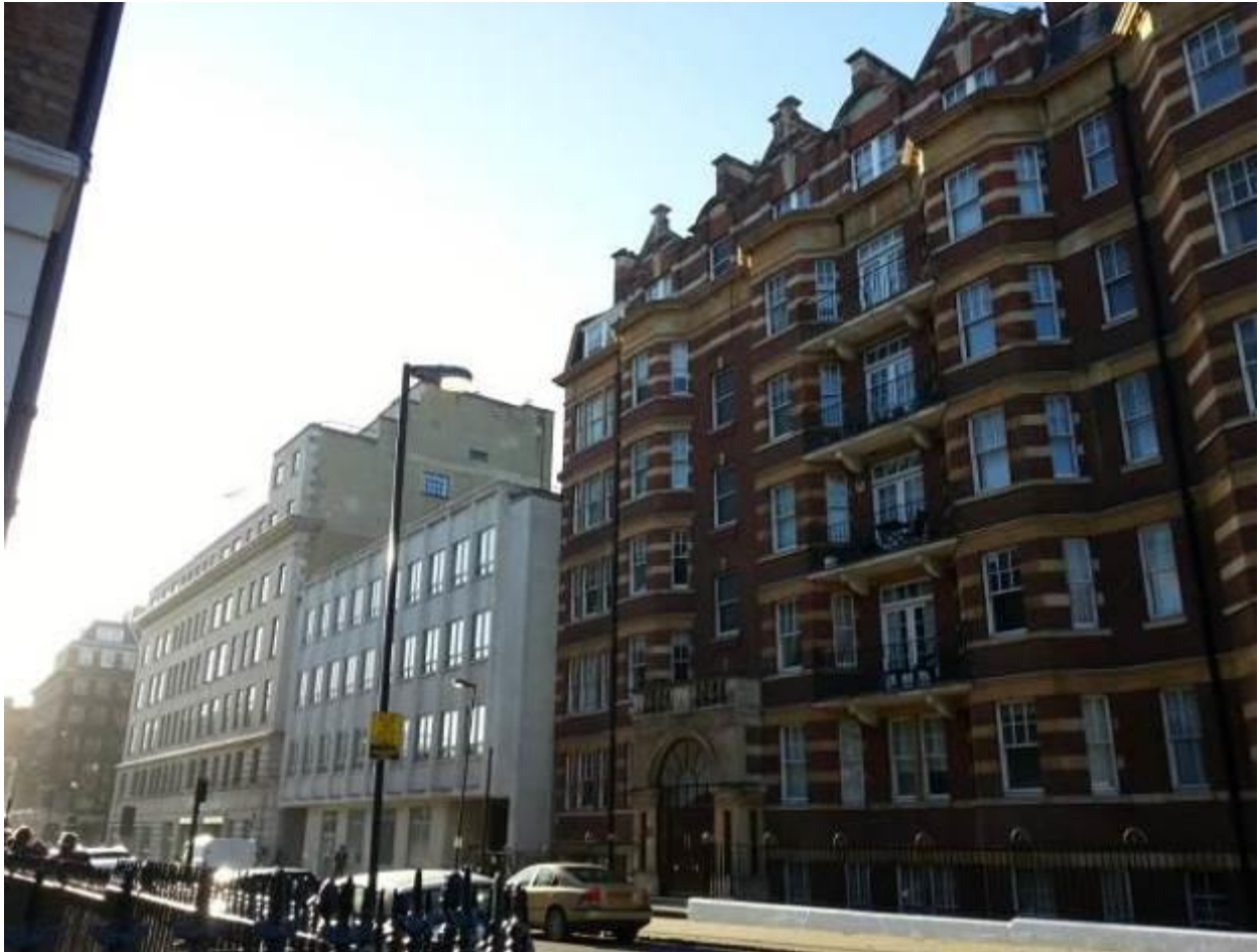
Application Site (left) from Balcombe Street. Melcombe Court to Right.
