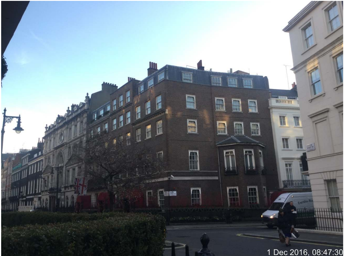
View of application site from street level (the corner of Charles Street and Queen Street)
